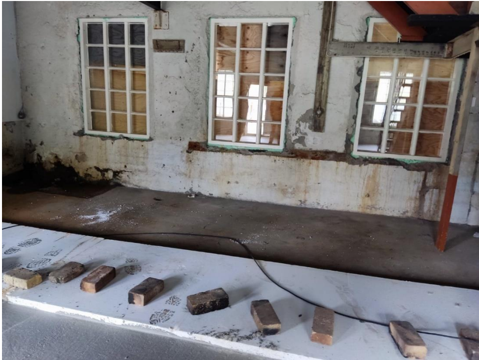
The inside of Tæknimínjasafn Austurlands premises are also under construction, Seyðisfjörður.
