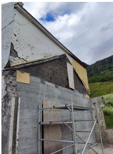
The new entrance of Tæknimínjasafn Austurlands under construction, Seyðisfjörður.
